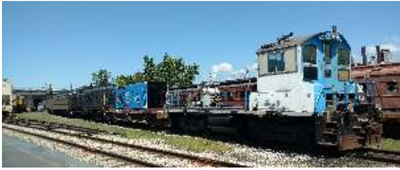
Sand blasting locomotive and passenger cars
