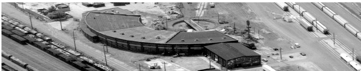
Cleveland's Historic B&O Roundhouse, circa 1970s, as it once stood with all stall sections intact
